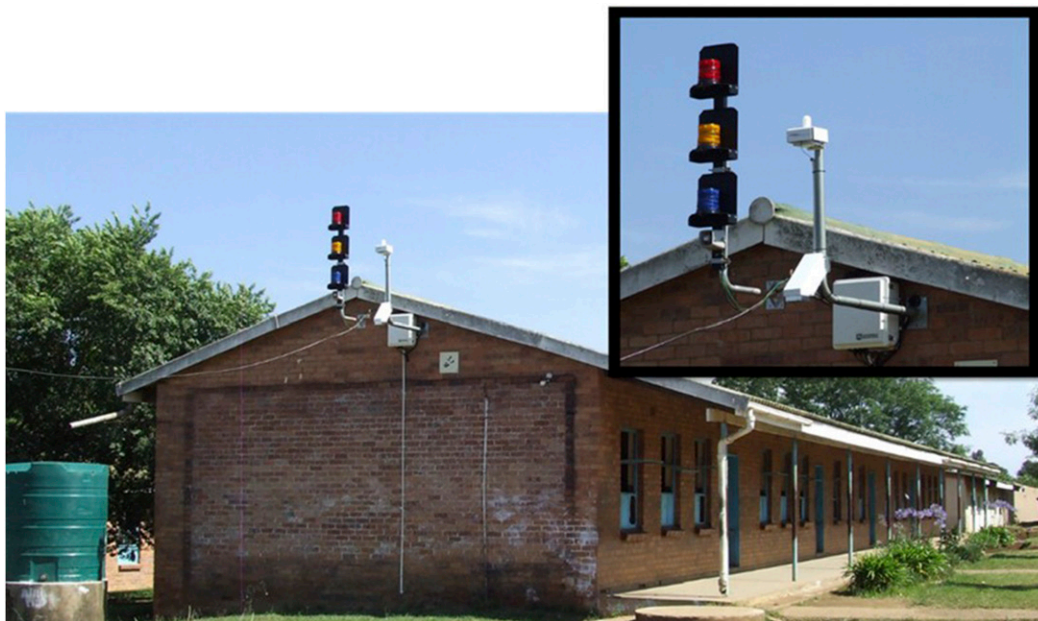
FIG. 2. The LWS located at the Swayimane High School, Swayimane. The CS110 EFM, the SG000 lightning flash sensor, the siren, and strobe beacon lights are visible in the inset image.
